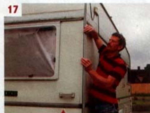
17 ■ Each section was pressed firmly into the bedding sealant, taking care to ensure there was continuity in the channelling groove
