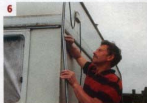
6 ■ A lower section was removed first and it was noted that some remnants were still in fairly good condition
