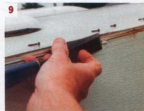
9 ■ An old blunt chisel was the only tool which would scrape away deposits of mastic
